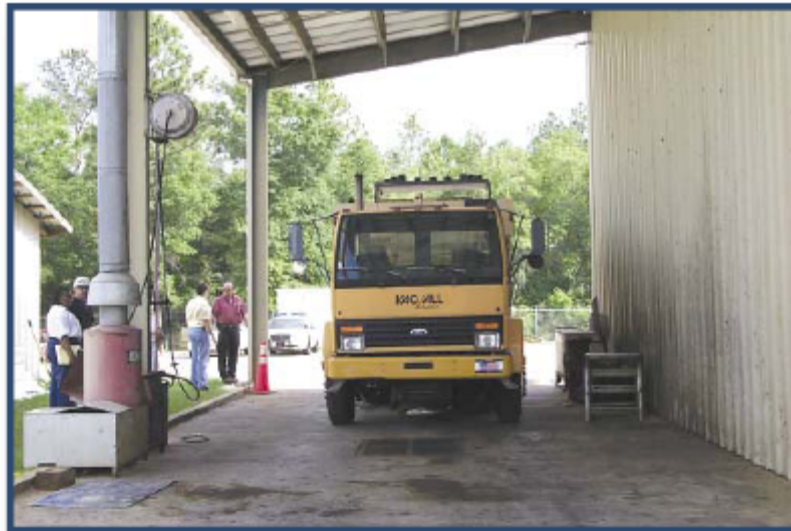
Figure 6. Truck wash facility, with open, roofed structure. The berm prevents the wastewater from running off the wash pad.
