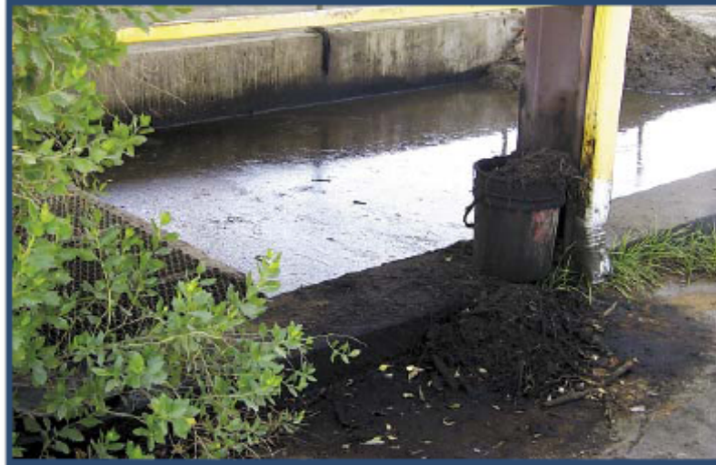
Figure 19. The solid waste collected from the settling pit is improperly stored in an open bucket. The waste should be stored in a closed container until ready to be sent to a class I or II sanitary landfill.
