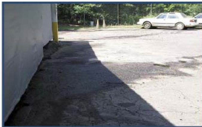
Figure 12. Outside view of the same facility. Because of the improper containment, the wash water runs outside, off premises, and onto the ground.
