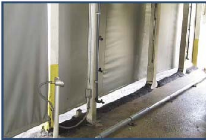
Figure 11. The gap between the overspray abatement curtains and the curb at this car wash facility allows wash water to escape outside the impervious area.
