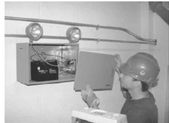
Remove Panel Door Fasteners
