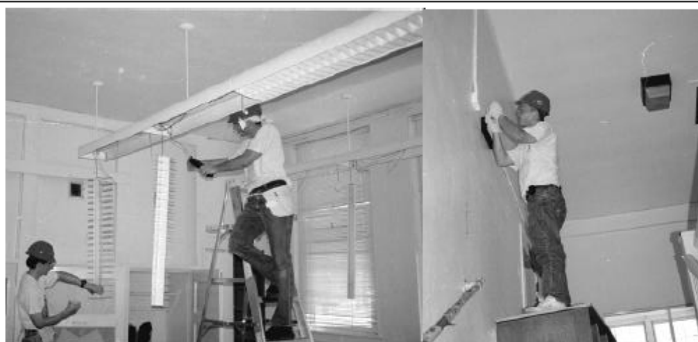
Removal of Small Sealed Lead Acid from Emergency Light
