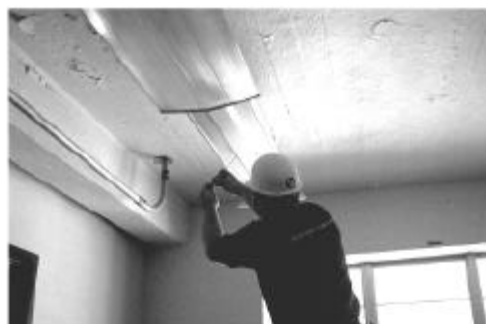
After removing bulb, remove ballast cover.
