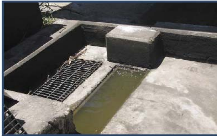
Figure 18. The wash pad at this facility is equipped with a stormwater diversion valve.
