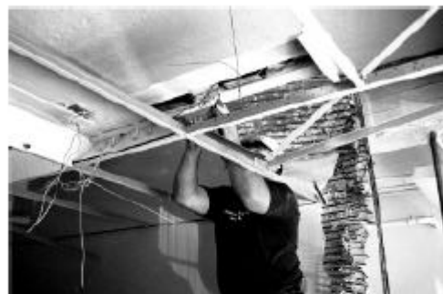
Remove restraining bolts.
