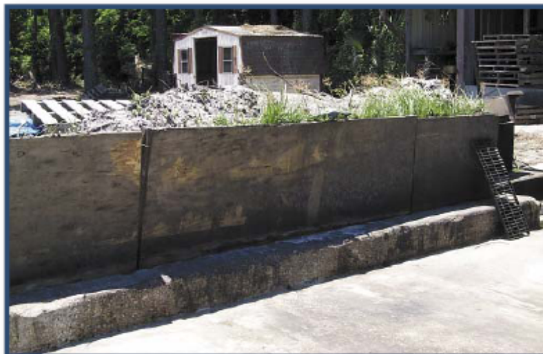
Figure 20. Example of improper storage of solids. The material is not completely covered and as a result, the rain water can wash it away.
