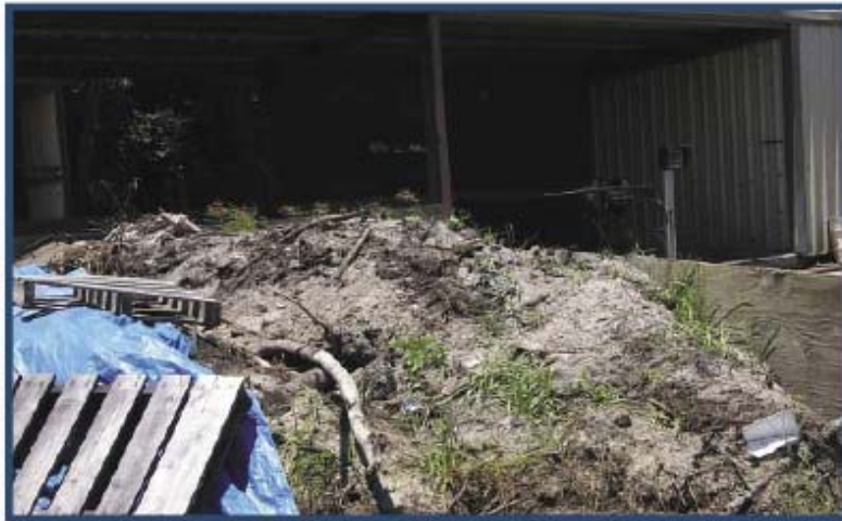
Figure 22. Example of improper handling of solids. Solids should be stored on an impervious surface, well covered, with no exposure to rain.
