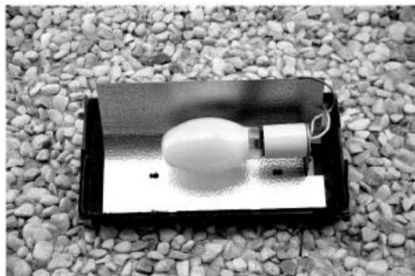
Remove cover to expose HID lamp
