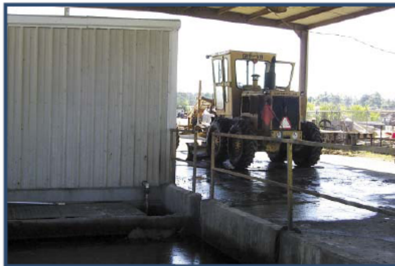
Figure 7. Covered concrete wash pad. Wastewater collects into the adjacent pit via the gate.
