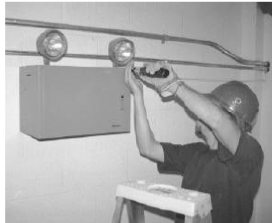
Remove Panel Door Fasteners
