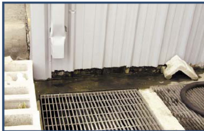
Figure 15. The collection pit at this car wash facility is located outside, adjacent to the wash tunnel. The pit is not covered, there is no overhang, and the downspout brings rain water right into the pit. This situation must be corrected.
