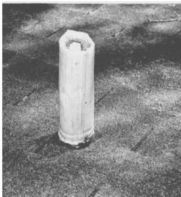
The durable and maleable properties of lead make it an excellent material for protecting and sealing pipes and vents on roofs.
