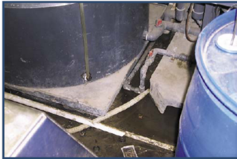
Figure 26. Scattered pieces of different materials in a puddle of liquid on the floor are signs of poor housekeeping. Poor housekeeping creates safety hazards, as well as operational problems.
