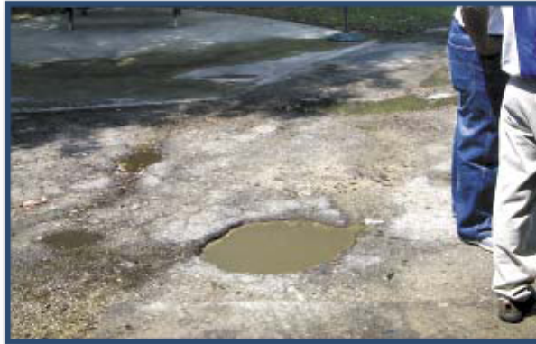
Figure 14. Dirty water in this puddle just outside the car wash tunnel indicates some car washing took place outside the wash tunnel, allowing dirty water to run onto the ground instead of into the collection pit.
