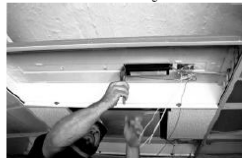
Cut wires and remove ballast.
