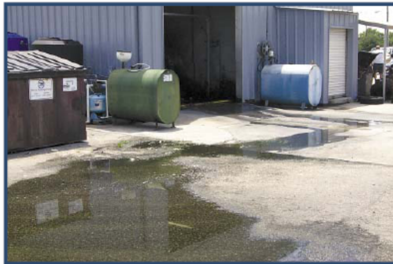
Figure 9. The rinse water at this car wash facility is allowed to collect on site, creating nuisance conditions.
