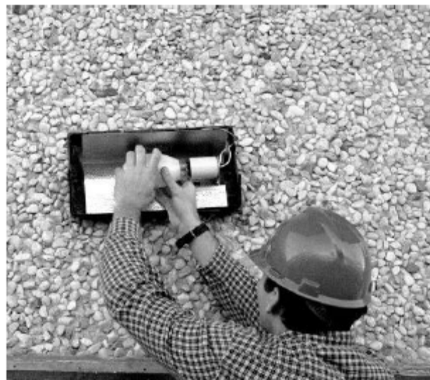
Remove cover to expose HID lamp
