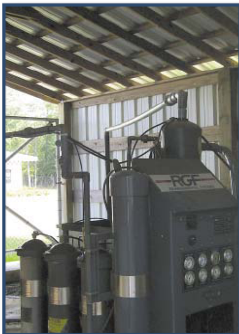
Figure 13. Example of a 100% closed-loop recycle treatment unit installed in an enclosed space to prevent rainwater from getting in, as well as, to prevent unwanted tampering with the control panel.
