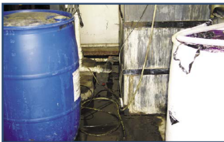
Figure 25. The recycling system at this facility is enclosed and it is therefore protected from stormwater intrusion. The liquid on the floor indicates a spill or leak. This situation must be corrected.
