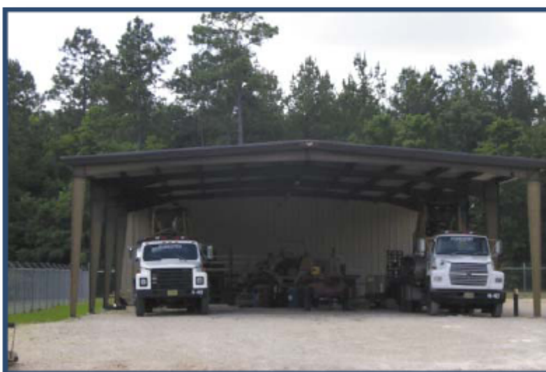
Figure 23. At this facility heavy equipment is completely covered for protection from the inclement weather, and also to prevent runoff contamination. If a roofed structure is not feasible, at least the dirty portions of the equipment should be covered.
