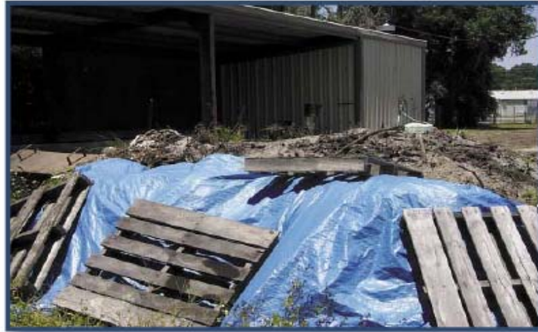
Figure 21. Example of improper handling/storage of solids. An attempt was made to cover the pile with a tarp; however the coverage is not complete, so the rain water can wash and carry away solids from the pile.
